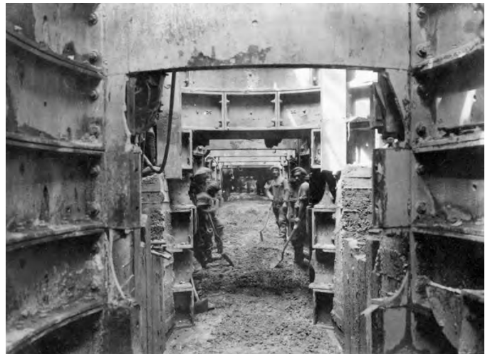
Tough and dangerous working conditions in the trench
