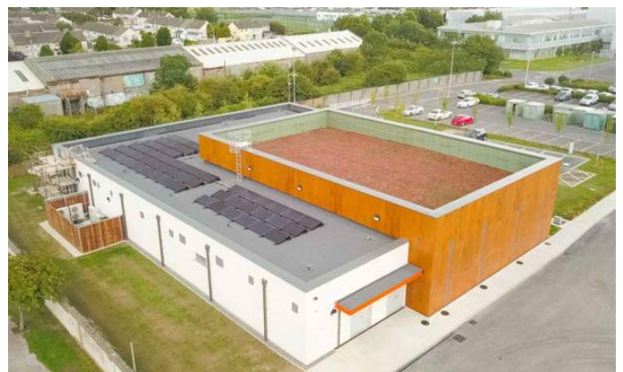
Solar panels supplement the buildings energy requirements.
